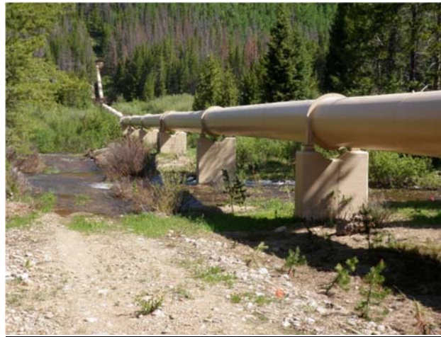
Part of siphon over wetlands in Jim Creek valley
