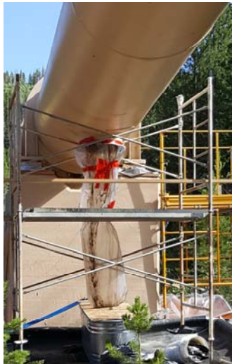
Spent lining waste funneled out of siphon
