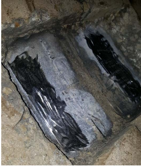
Figure 2. Exposed & Cleaned Joint
