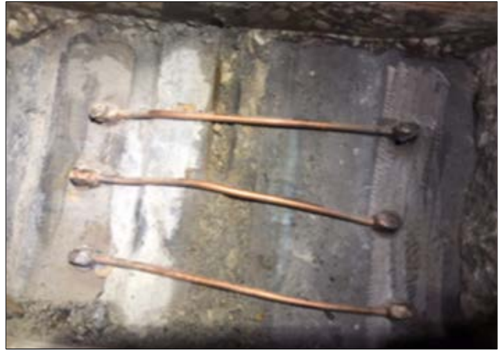
Figure 3. No.4 AWG Wires Thermite Welded
