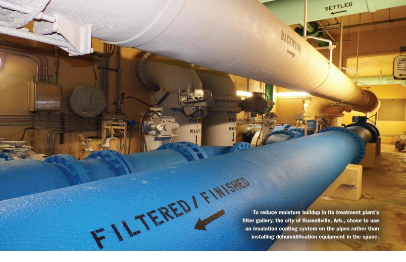
coating by removing loose rust and previous coatings. They were then coated with a one-component, micaceous iron oxide- and zinc-filled primer, Tnemec's Series 394 PerimePrime. By applying a high-performance primer, the pipes were protected from other common corrosion problems for years to come, thanks to a triple-barrier mechanism of zinc, micaceous iron oxide, and urethane.
